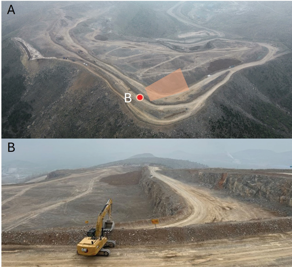
Figure 6-2: Quarry current conditions
