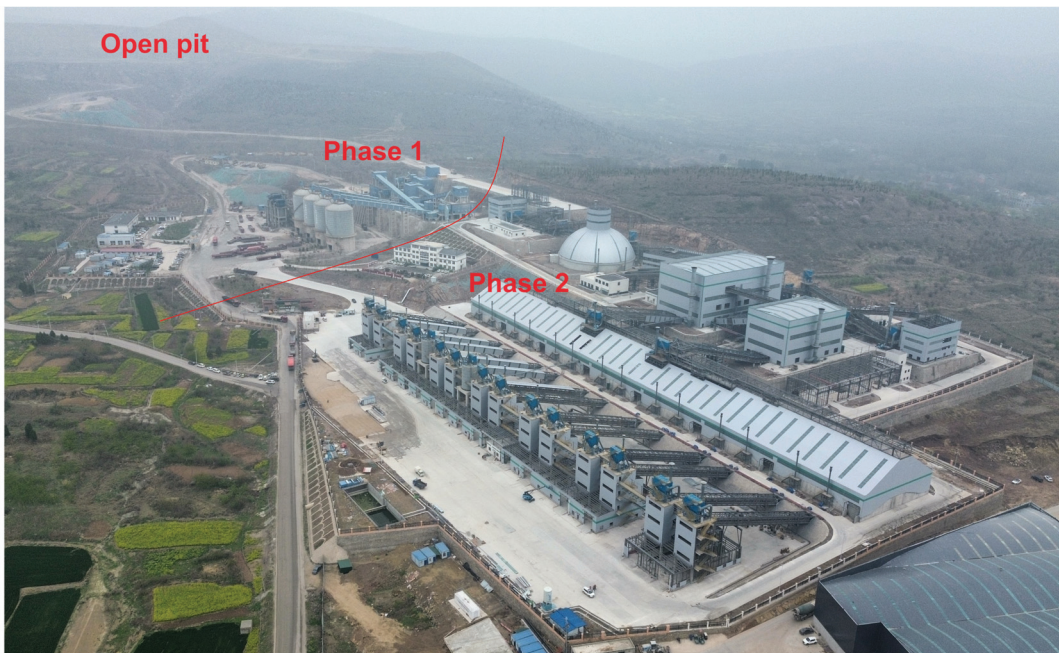
Figure 8-1: Existing and proposed approximate location of the Phase II processing plant, looking east
