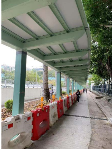
Construction of Walkway Cover
