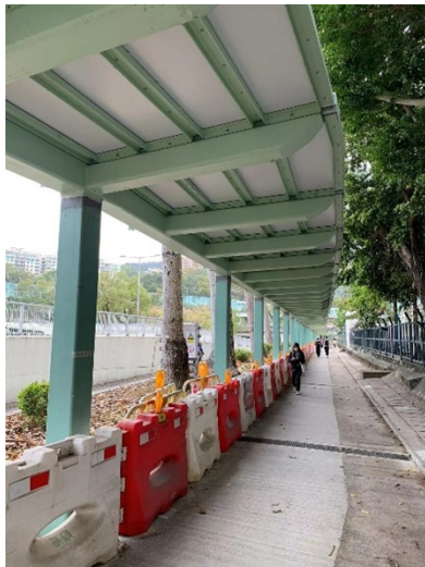
Construction of Walkway Cover
