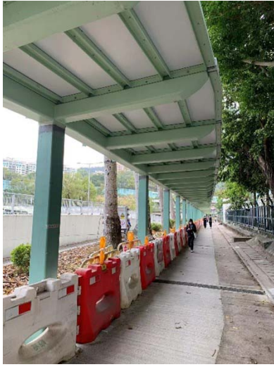
Construction of Walkway Cover
