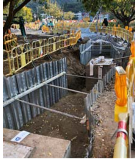
Construction of Sewage System
