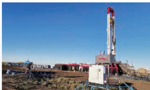
Drilling rig for new wells drilling
