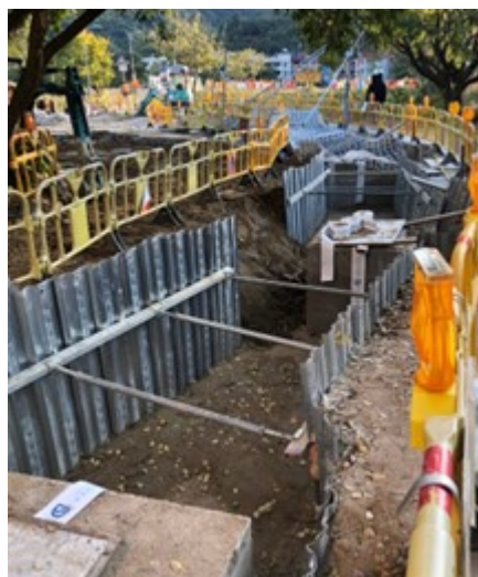
Construction of Sewage System
