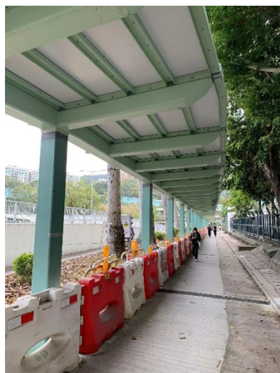
Construction of Walkway Cover
