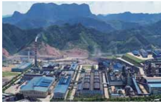
Key technologies and equipment for the coordinated smelting and comprehensive recovery of lead, antimony and silver multi-metal materials
