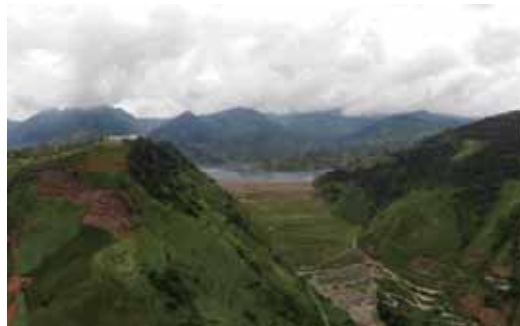
Key technologies for tailings dam survey and its early warning and disaster control evaluation
