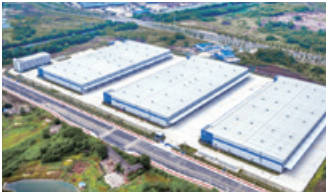
34 Chongqing Shuangfu Project
