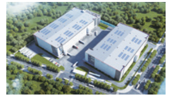
12 Nanjing Jiangning Project#
