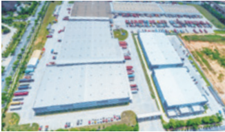
8 Shenzhen Pingshan East Project
