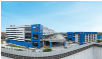
12 Foshan Nanhai Project
