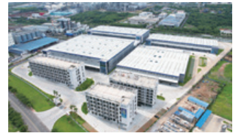
41 Hainan Yangpu Project
