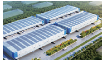
14 Foshan Gaoming Project#
