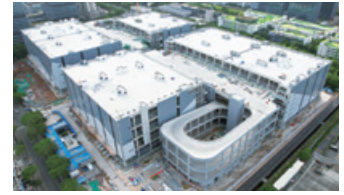
7 Shenzhen Pingshan Project
