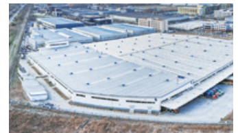
20 Tianjin Binhai Project
