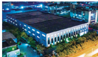
6 Shanghai Qingpu Project
