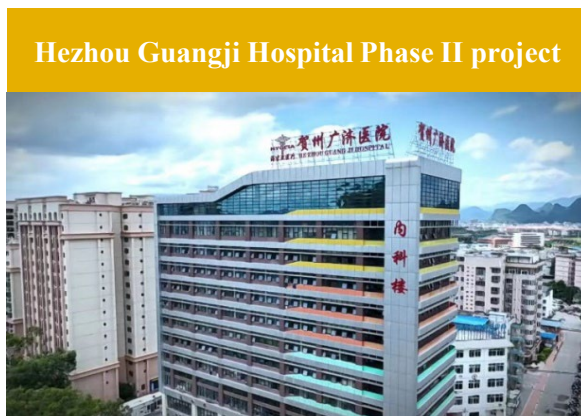
The preparation works of the Hezhou Guangji Hospital Phase II project has commenced Expected to additionally accommodate approximately 500 beds when it commences operations
