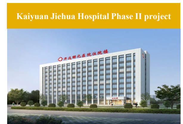
Kaiyuan Jiehua Hospital Phase II project has commenced civil engineering construction Expected to additionally accommodate approximately 500 beds when it commences operations
