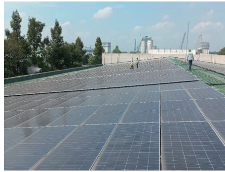
Maintenance of solar PV panel in Vietnam factory
