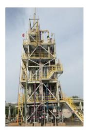
We use the "two-stage CLAUS + selective hydrogenation + selective oxidation" process, with a total sulfur recovery rate above 99%.
