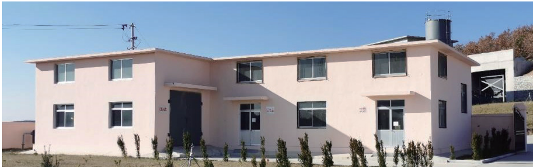
壓縮空氣及配電樓
