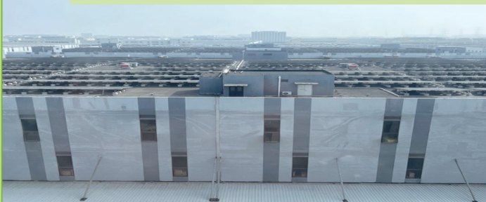
■ Logistics centers fully covered with rooftop PV
