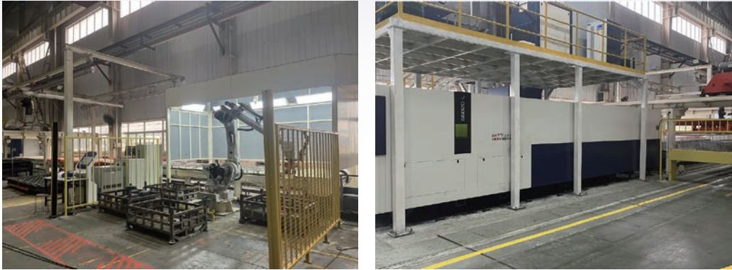
Cutting Noise Reduction Transformation Project of Dongfeng Liuzhou Motor
