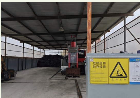
Hazardous waste storage
