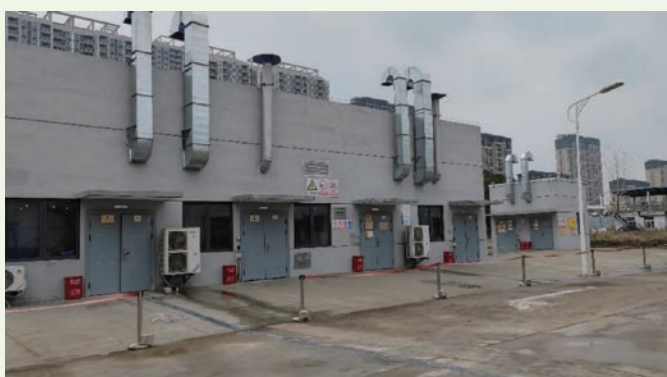
Dongfeng Motor Group Thomson Carbon Canister Laboratory Construction and Factory Relocation Project
