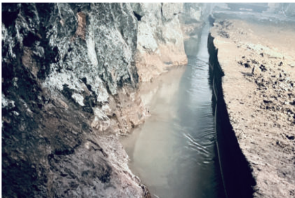
Kinsenda礦場巷道排水溝 Drainage Ditch at Kinsenda Mine
