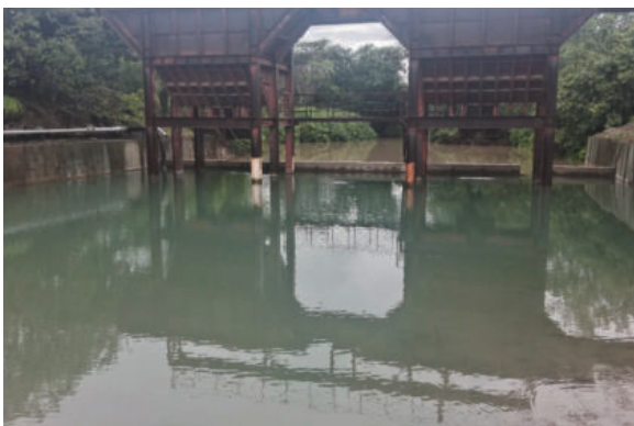
Kinsenda礦場地表蓄水池 Surface Drainage Reservoir at Kinsenda Mine
