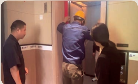
Rescue operations by maintenance officers
