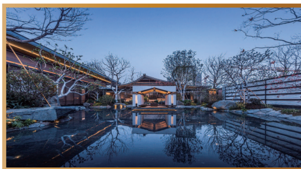
Real-site Photo of “Zen Chinese (禪境中式)” Architecture (Suzhou Tanfu* (蘇州檀府))
