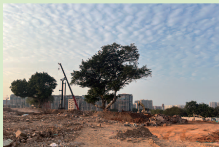
Century-old banyan tree at Wuyuan Bay* (五緣灣海)
