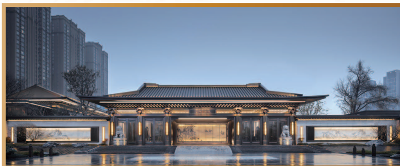
Real-site photo of “Emperor Chinese (王府中式)” Architecture (Chengdu Yangxi* (成都央玺))
