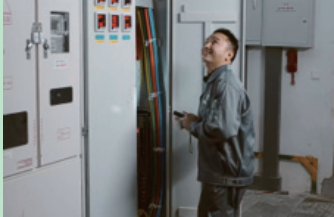
Photo of after-sales inspection
