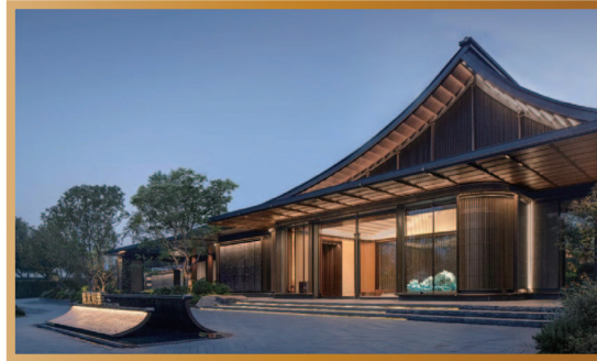
Real-site Photo of “Shiyi Dongfang (詩意東方)” Architecture (Suzhou Langyun* (蘇州朗雲))
