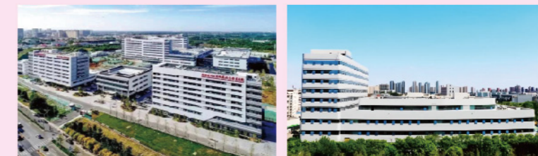
Some projects under management of Capital Jiaye (from left to right: Anzhen Hospital, Guang'anmen Hospital)
