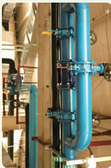
Renovation of the cooling water tower in Building G G棟冷卻水塔改造
