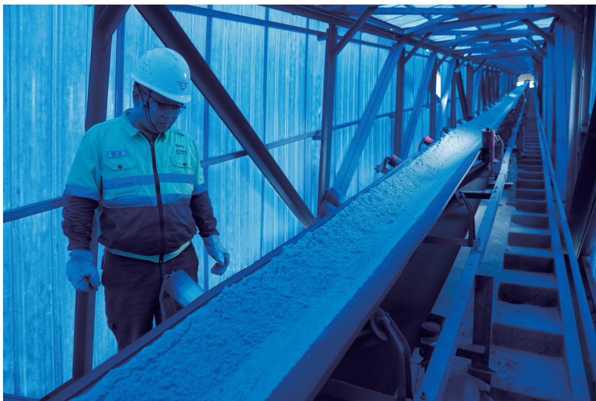
Lithium concentrate production line
