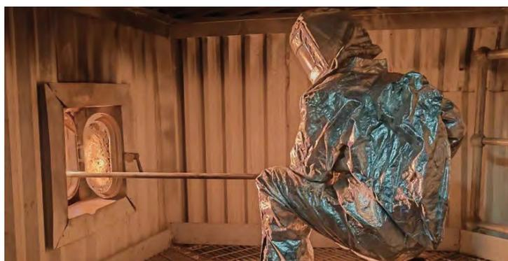
Centralized control inspector performed boiler fire inspection and slag cleaning
