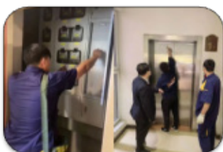
Outage and lock ladder 斷電、鎖梯
