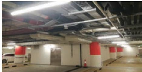
12,000 sets of existing double fluorescent lights in the car park were replaced with LED tubes. Out of these, 400 sets were replaced with motion sensor-enabled single 18W LED tubes. We have also replaced 580 compact downlights in the back of house corridor with all-in-one LED downlights.
