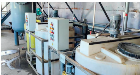
氣浮機改造 Steam floatation machine upgrading
