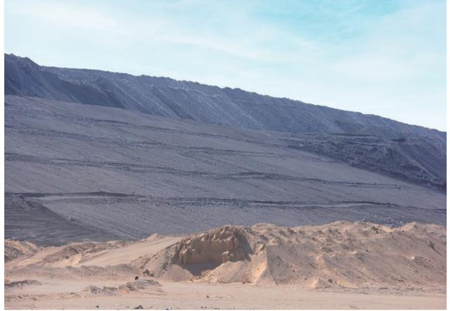
During technical rehabilitation: Covering topsoil on the shaped waste piles.
