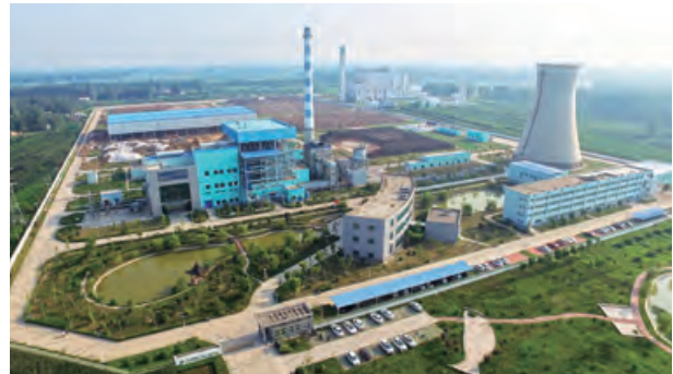
Dangshan Integrated Biomass and Waste-to-energy Project 蕩山生物質及垃圾發電一體化項目
