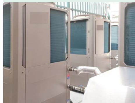
In addition to energy innovation and optimization in production regions, the Group also focuses on energy efficiency in non-production regions. In 2023, we pilot the Air Energy Water Heater for dormitories, heating the water through the valley electricity. Through the pilot, found that the consumption of air energy water heaters is more energy efficient than traditional outsourced steam heating, saving about 30% of energy use compared to the previous period.
