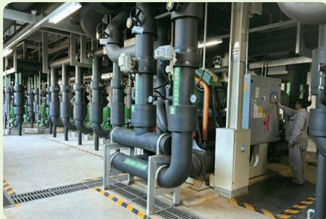
Daxing branch factory’s ground source heat pump system
