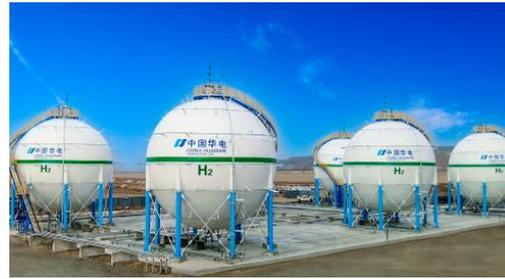
Hydrogen Gas Storage Tanks of Huadian Green Hydrogen Demonstration Project
