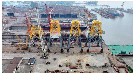
The World's First "Integrated Equipment of Foundation Jacket for Wind Turbines + Net Cage"
