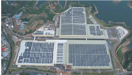
均州工廠三期光伏屋頂俯瞰圖 Aerial View of Phase III Rooftop Photovoltaic Power Generation System of Junzhou Factory
