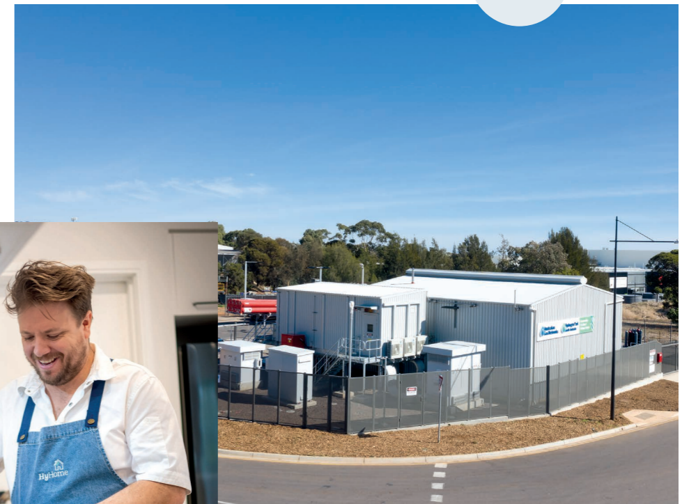
AGIG's Hydrogen Park facility in South Australia.
