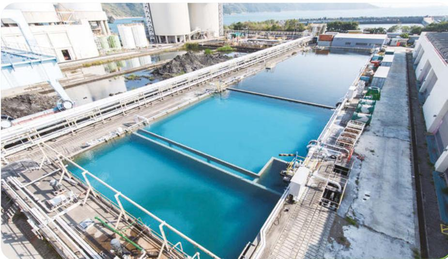
We treat our wastewater in accordance with local regulations to remove oil, grease, suspended solids and heavy metals, and we disinfect our treated effluent discharge from the on-site sewage treatment plant using ultraviolet technology systems. We also monitor discharge of effluents in accordance with local licensing requirements. In 2023, 100% of the effluent discharged from LPS satisfied those requirements.
