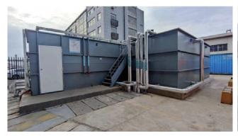
The sewage treatment station in Lianyungang New Oriental Terminal is used to treat and purify the sewage to achieve the discharging standard or reuse.
