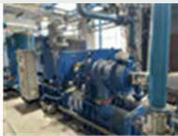
Air compressor residual heat recovery unit
