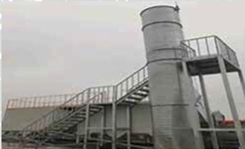
Injection moulding exhaust treatment system
