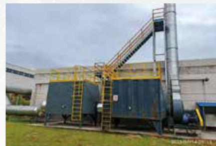
Two-stage activated carbon adsorption treatment equipment
