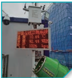
Example of environmental monitoring system
