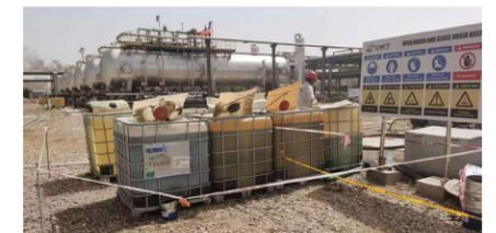
Recycling areas on CPF stations with material bags and chemical bins to prevent waste oil from causing soil contamination and realize resource recycling and reutilization
