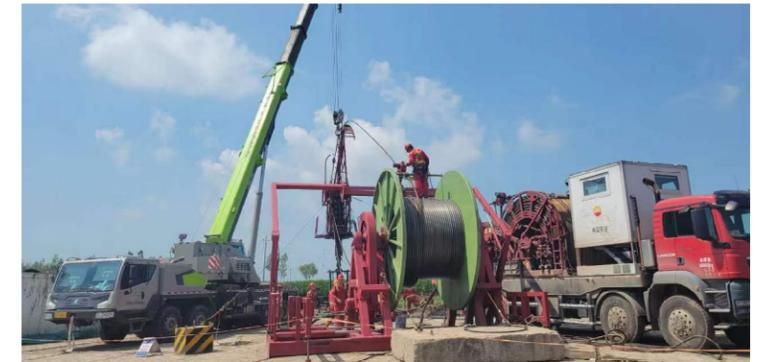
Anton achieved the world's first application of fiber-optic monitoring technology in a U-shaped geothermal well, providing clients with data support for the exploitation of renewable geothermal energy
