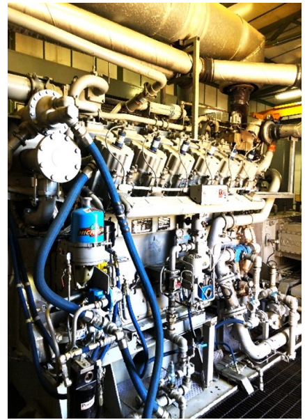
Part of the newly acquired RGP – low pressure gas is compressed to sales gas pressure using gas engine driven reciprocating compressors
