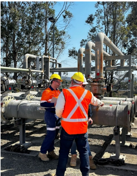
Part of the newly acquired RGP - Gas will be delivered to the Carpentaria Gas Plant via the buried gas gathering system at low pressures to maximise well deliverability
