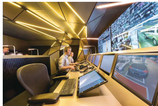
Car park operations and facilities management
