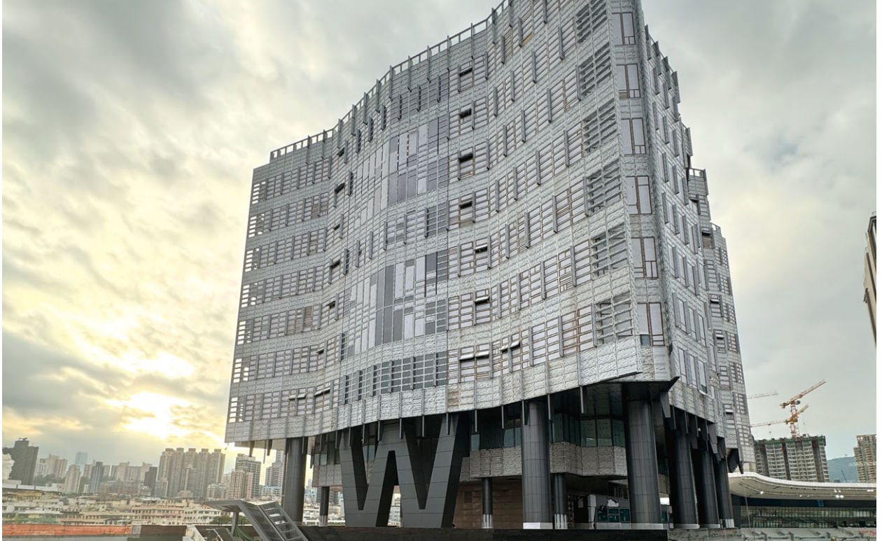
Hong Kong Kai Tak Development – Office
