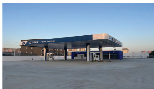
Zhengzhou High-Tech Industrial Development Zone hydrogen gas station
