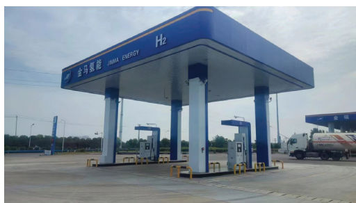
Jiyuan High-Tech Industrial Chemical Park hydrogen gas station
