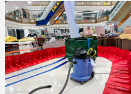
Use 660-litre bin and submersible pump to drain water
