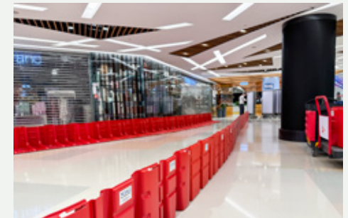
Install flood barriers and sandbags for flood control
