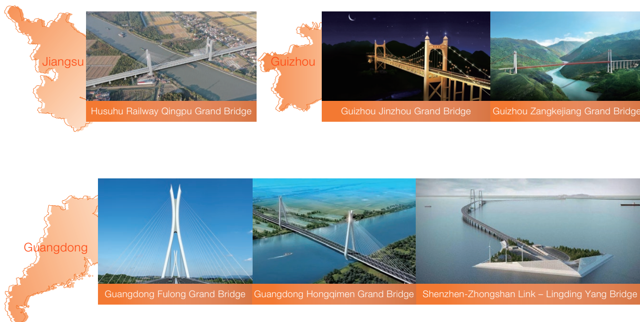
Photos of on-going projects for the Cable Business
