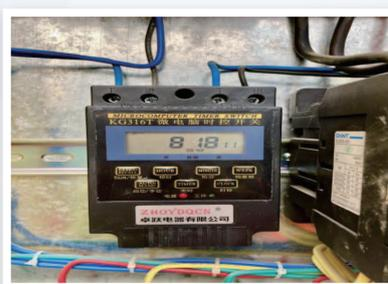
**Distribution boxes equipped with time switches**
