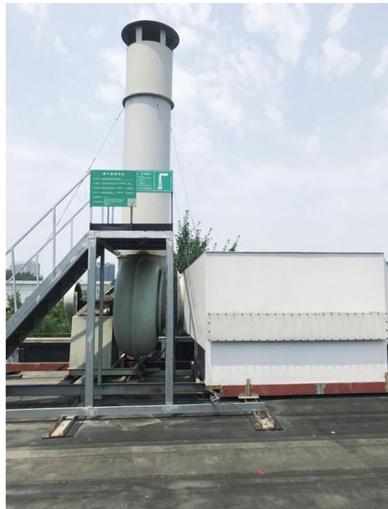
Activated Carbon Adsorption Device
