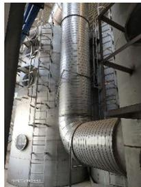
Spraying Tower for handling of paint exhaust
