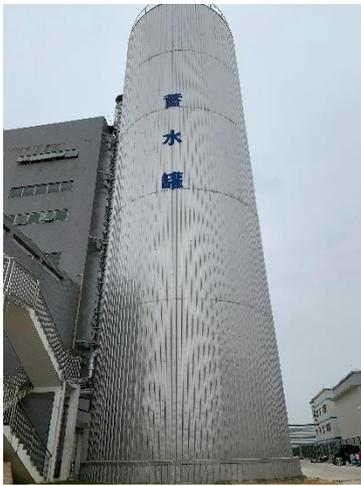
Water Storage Tank – cold energy storage / air-conditioning equipment
