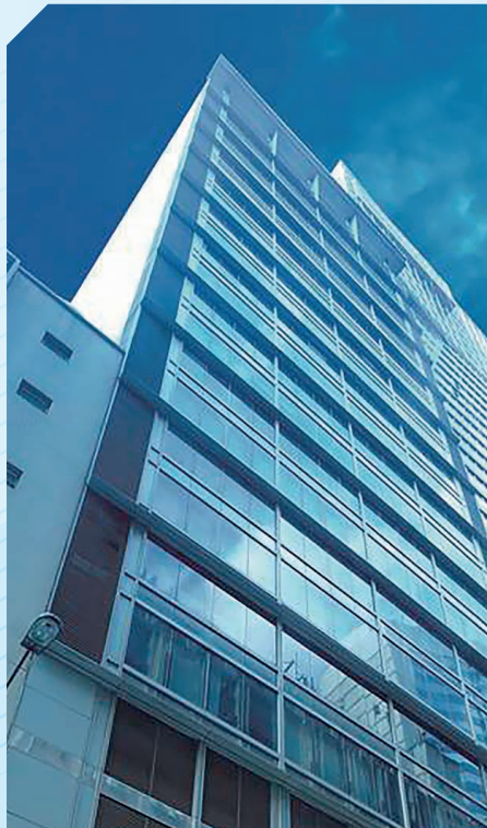
9 CHONG YIP STREET
