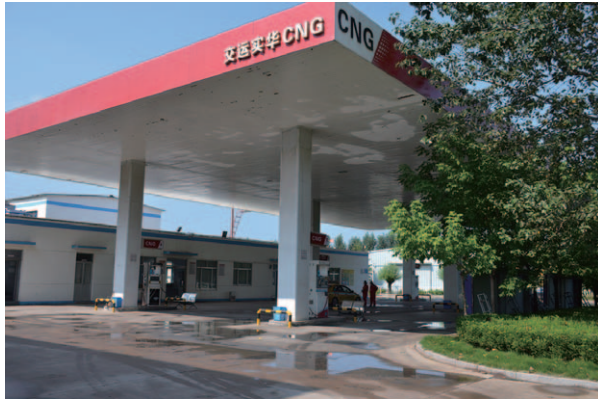
No. 1 Refuelling Station
