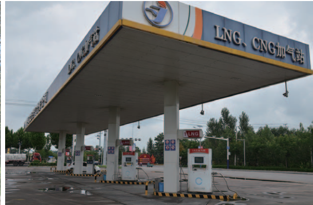
Longtan Road LNG and CNG Refuelling Station
