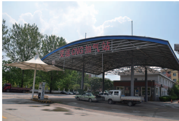
No. 2 Refuelling Station
