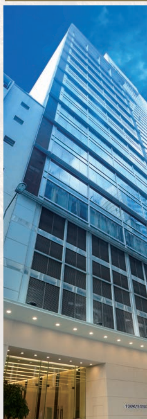
9 CHONG YIP STREET
