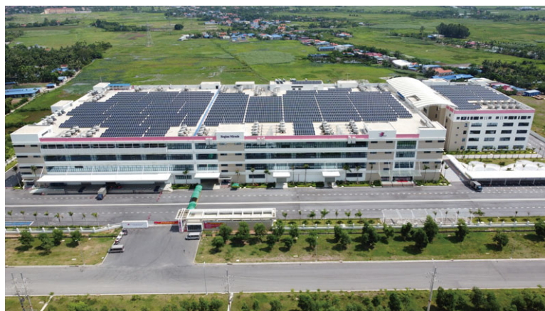
Roof solar panel system of the Vietnam factories 越南廠區屋頂太陽能電池板系統
