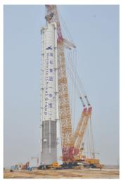
One of the key equipment in the Chemical propane dehydrogenation device (PDH device), the rectification tower for separating the mixture of propane and propylene, the diameter exceeds 10 meters, and the length exceeds 120 meters.
