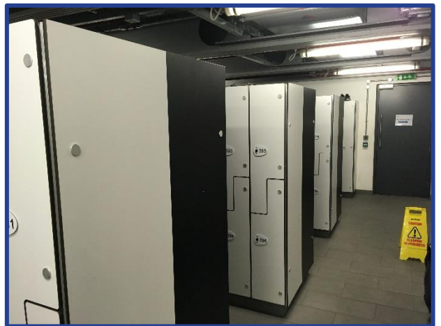
Shower and Locker Facilities
